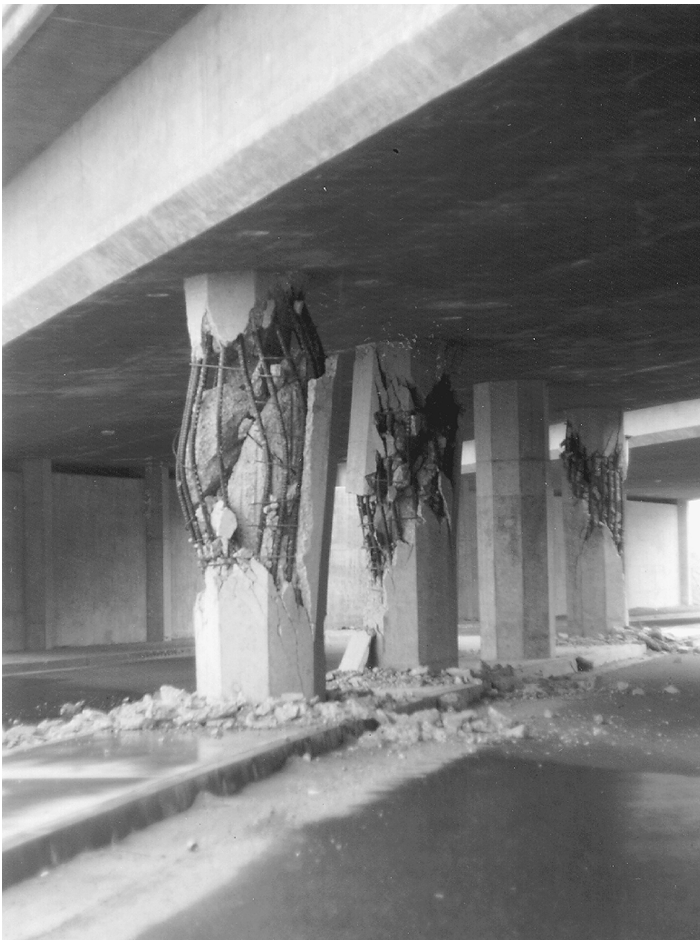
FIGURE 2.20 Failure of columns of the Route 5/210 interchange during the 1971 San Fernando earthquake.
