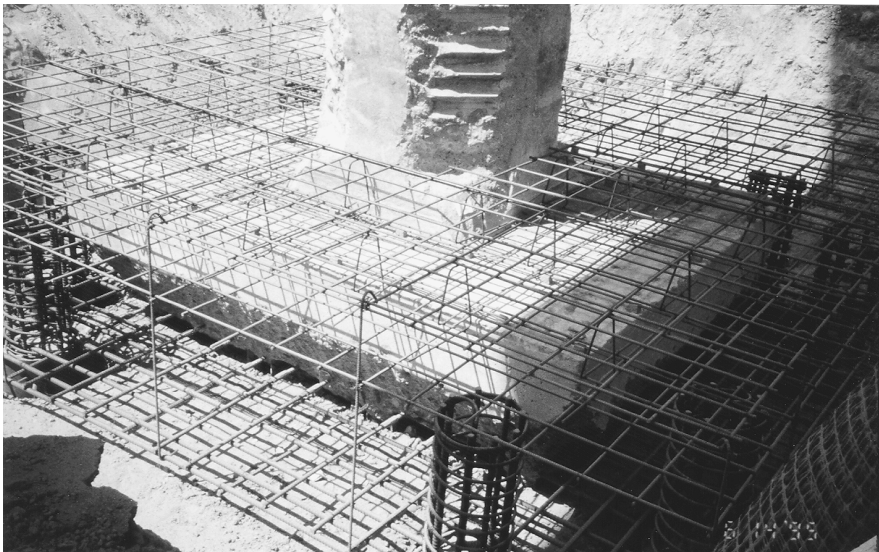
FIGURE 8.16 Typical footing and pile cap modification.
