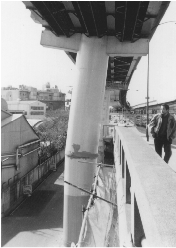
FIGURE 2.25 Local buckling of a circular cross-section column of the Hanshin Expressway in the 1995 Hyogo-Ken Nanbu earthquake.
