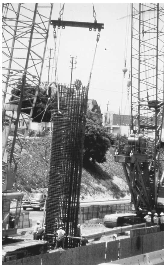
FIGURE 8.11 Column-reinforcing steel cage.
