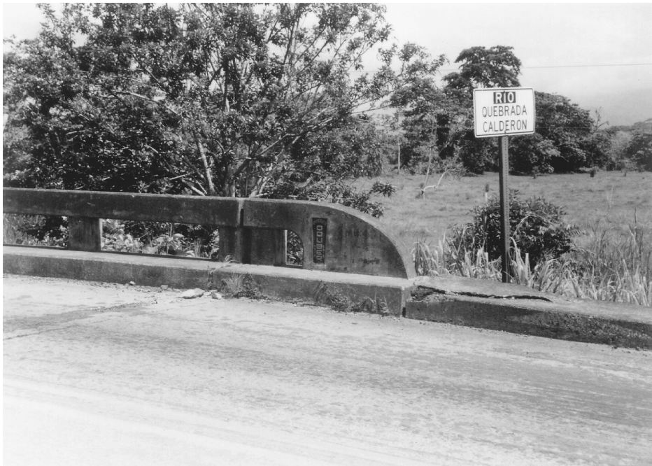
FIGURE 2.34 Settlement slab spanning across slumped abutment fill material at the Rio Quebrada Calderon bridge in the 1991 Costa Rica earthquake. (Source: EERI, Earthquake Spectra , Special Suppl. to Vol. 7, 1991.)
