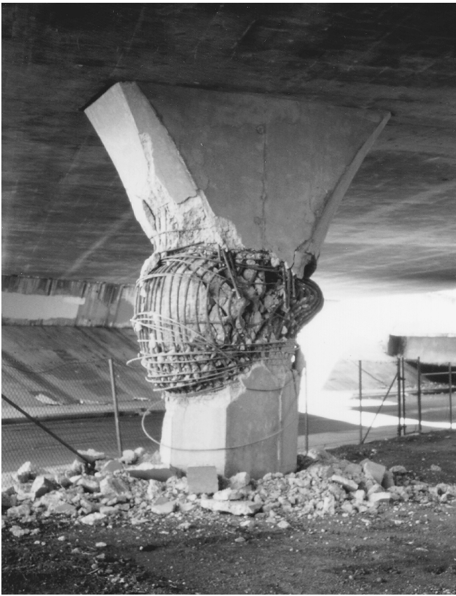
FIGURE 2.22 Failure of flared column in the Route 118, Mission-Gothic Undercrossing, in the 1994 Northridge earthquake.
