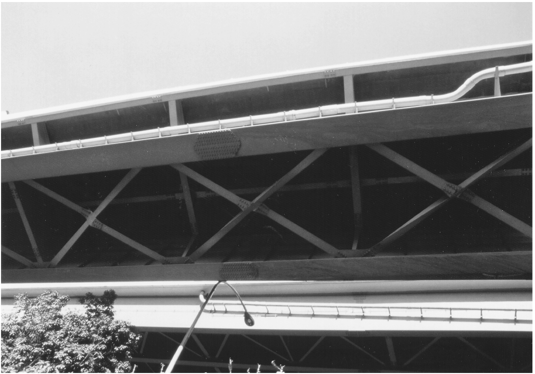
FIGURE 2.12 Buckling of braces near Pier 209 of the Hanshin Expressway in the 1995 Hyogo-Ken Nanbu earthquake.
