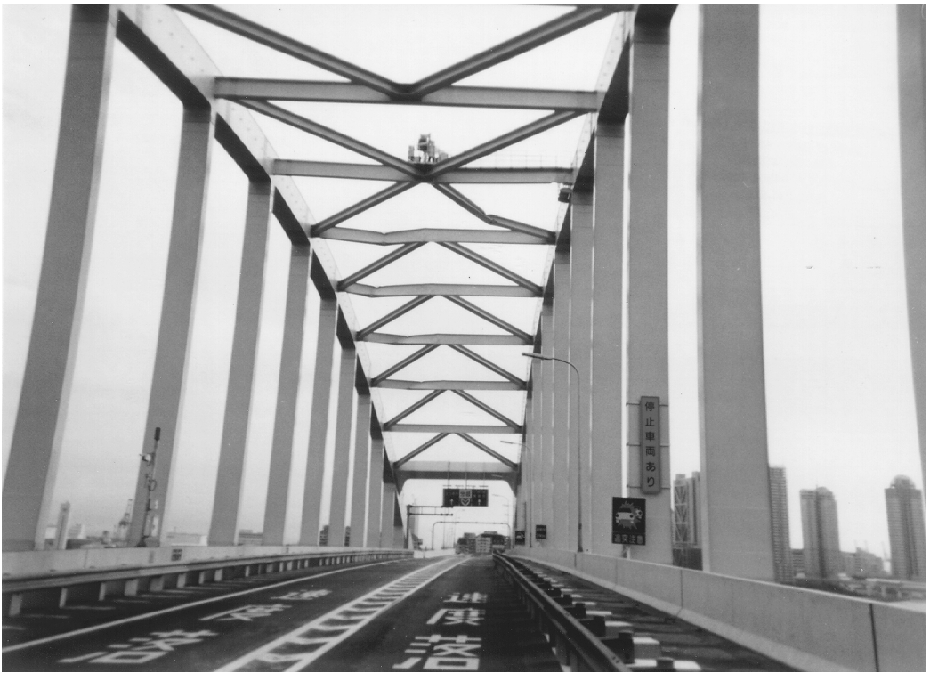
FIGURE 2.14 Buckling of cross-members in the upper chord of the Rokko Island Bridge in the 1995 Hyogo-Ken Nanbu earthquake.
