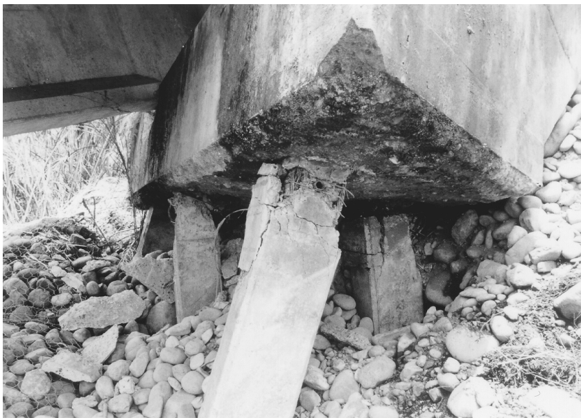
FIGURE 2.33 Abutment piles damaged during the 1991 Costa Rica earthquake. (Source: EERI, Earthquake Spectra , Special Suppl. to Vol. 7, 1991.)
