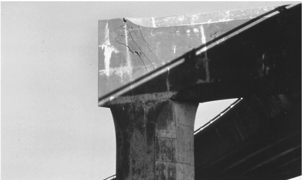
FIGURE 2.27 Outrigger damage in the 1989 Loma Prieta earthquake.
