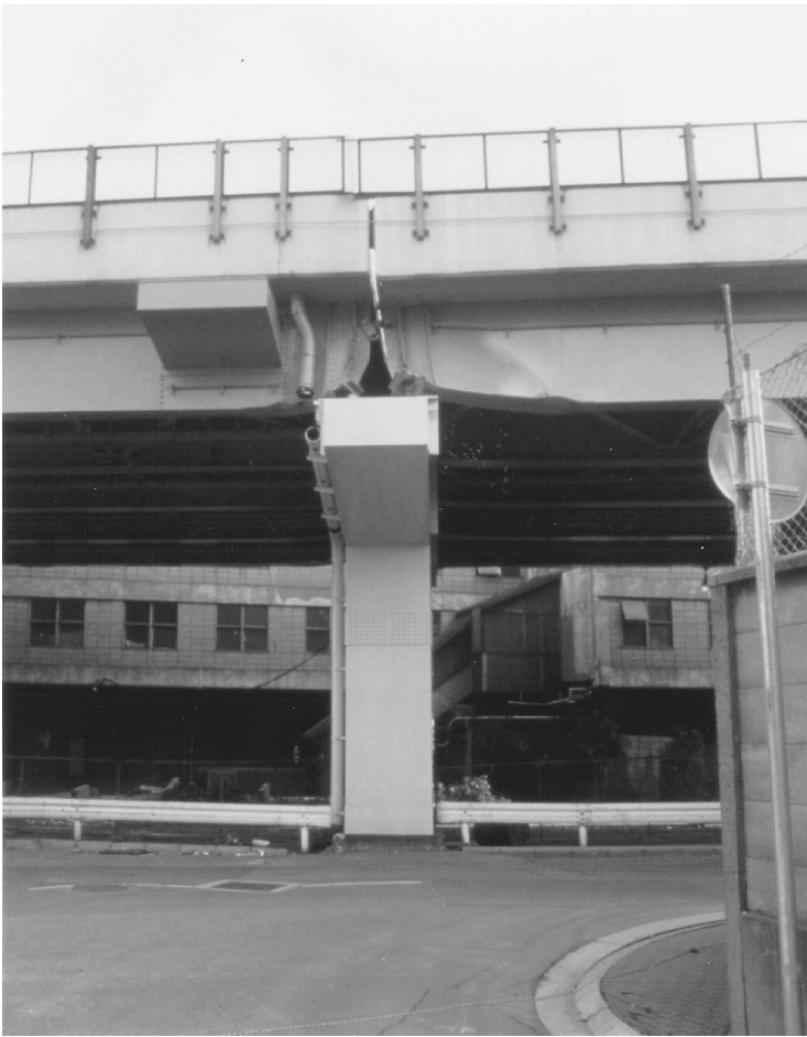
FIGURE 2.13 Girder damage at Bent 351 of the Hanshin Expressway apparently due to transverse movement during the 1995 Hyogo-Ken Nanbu earthquake.
