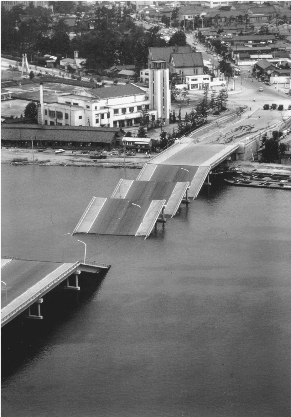
FIGURE 2.8 Showa Bridge collapse in 1964 Niigata earthquake.
