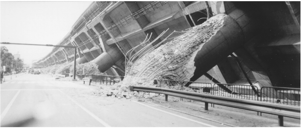
FIGURE 2.4 Higashi-Nada Viaduct collapse in the 1995 Hyogo-Ken Nanbu earthquake. (Source: EERI, The Hyogo-Ren Nambu Earthquake, January 17, 1995, Preliminary Reconnaissance Report, Feb. 1995.)
