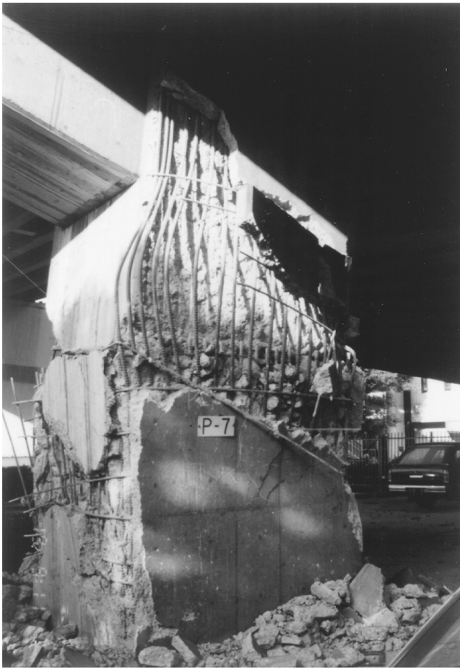
FIGURE 2.19 Failure of column with longitudinal reinforcement cutoffs near midheight in the 1995 Hyogo-Ken Nanbu earthquake.
