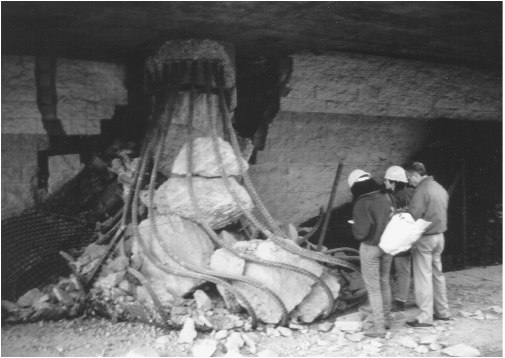
FIGURE 2.21 Failure of columns of Interstate 10, La Cienega-Venice Undercrossing in the 1994 Northridge earthquake. (Masonry walls of storage units are supporting the collapsed frame.)
