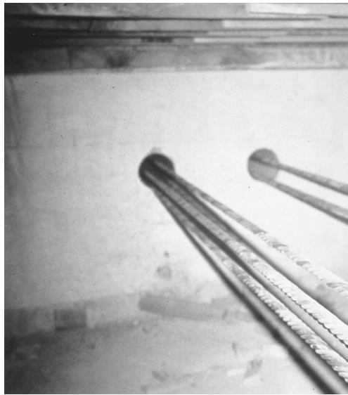
FIGURE 8.3 Hinge joint restrainer.
