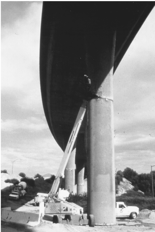
FIGURE 8.8 Steel jacket column retrofit.
