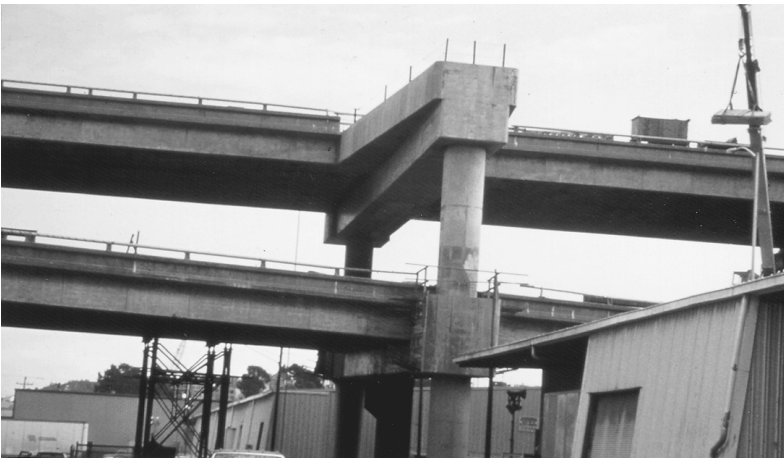
FIGURE 8.14 Completed retrofitted structures.
