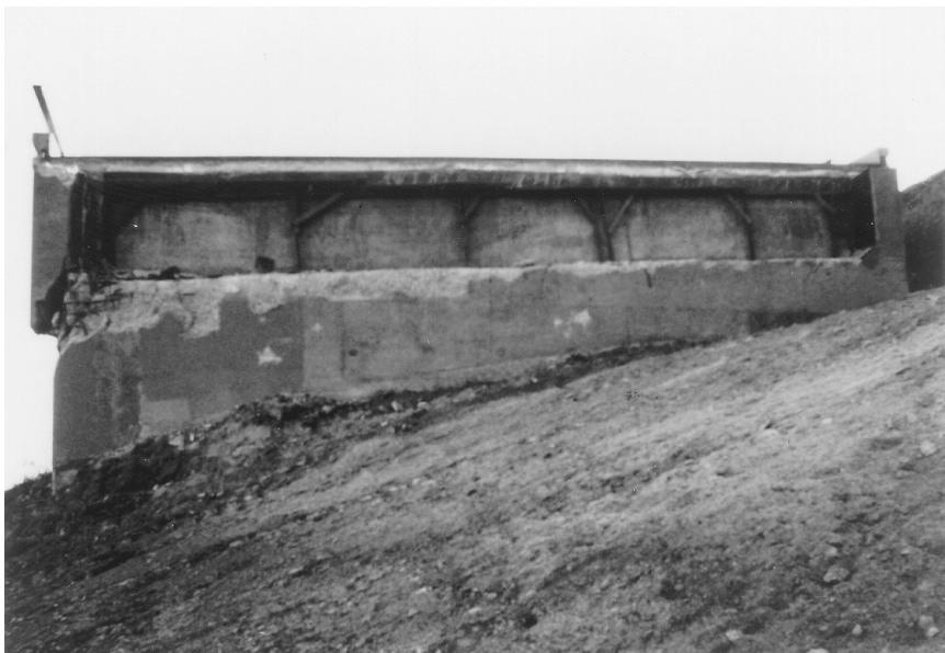
FIGURE 2.30 Damage to external shear key in an abutment in the 1994 Northridge earthquake. (Source: EERI, Earthquake Spectra , Special Suppl. to Vol. II, 1995.)
