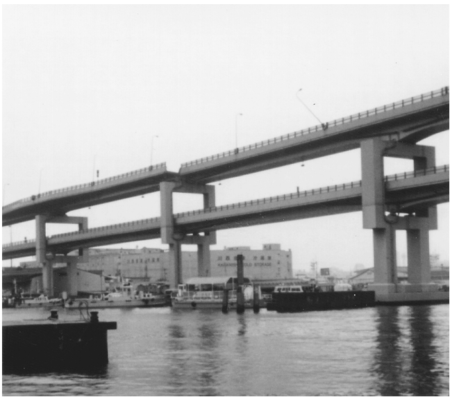
FIGURE 2.15 Hamate Bypass superstructure rotations as a result of bearing failures in the 1995 Hyogo-Ken Nanbu earthquake.
