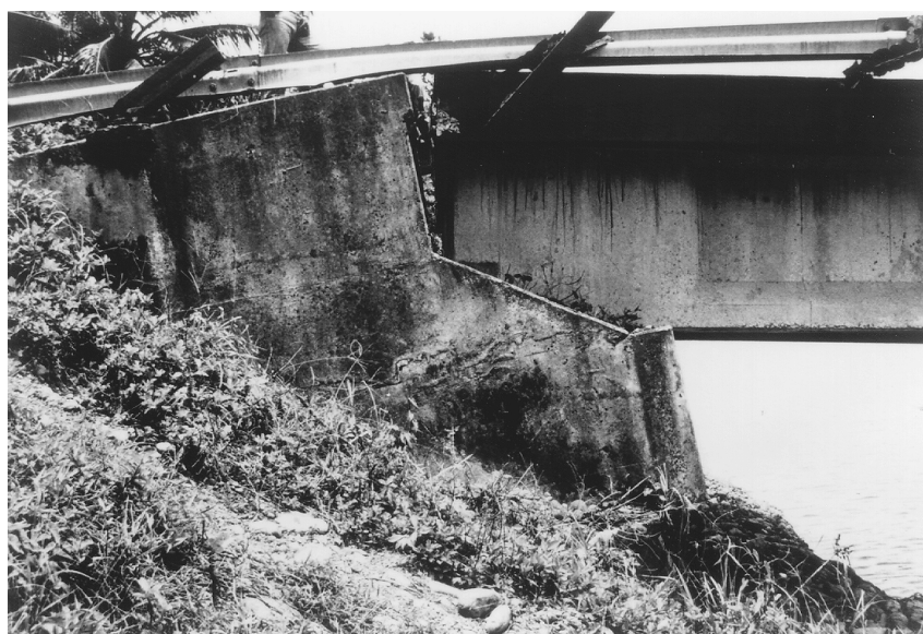
FIGURE 2.32 Rotation of abutment due to liquefaction and lateral spreading during the 1991 Costa Rica earthquake. (Source: EERI, Earthquake Spectra , Special Suppl. to Vol. 7, 1991.)
