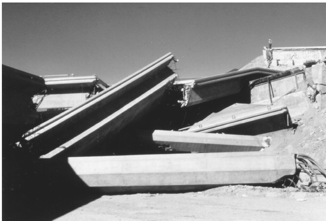
FIGURE 2.24 Failure at the base of a column supported on a single cast-in-place pile in the 1971 San Fernando earthquake (Steinbrugge Collection, EERC Library, University of California, Berkeley).
