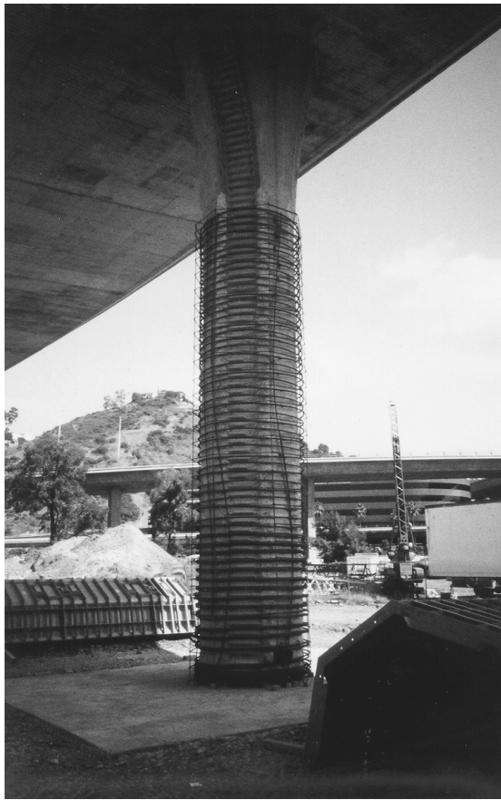
FIGURE 8.6 Reinforcement confinement retrofit.
