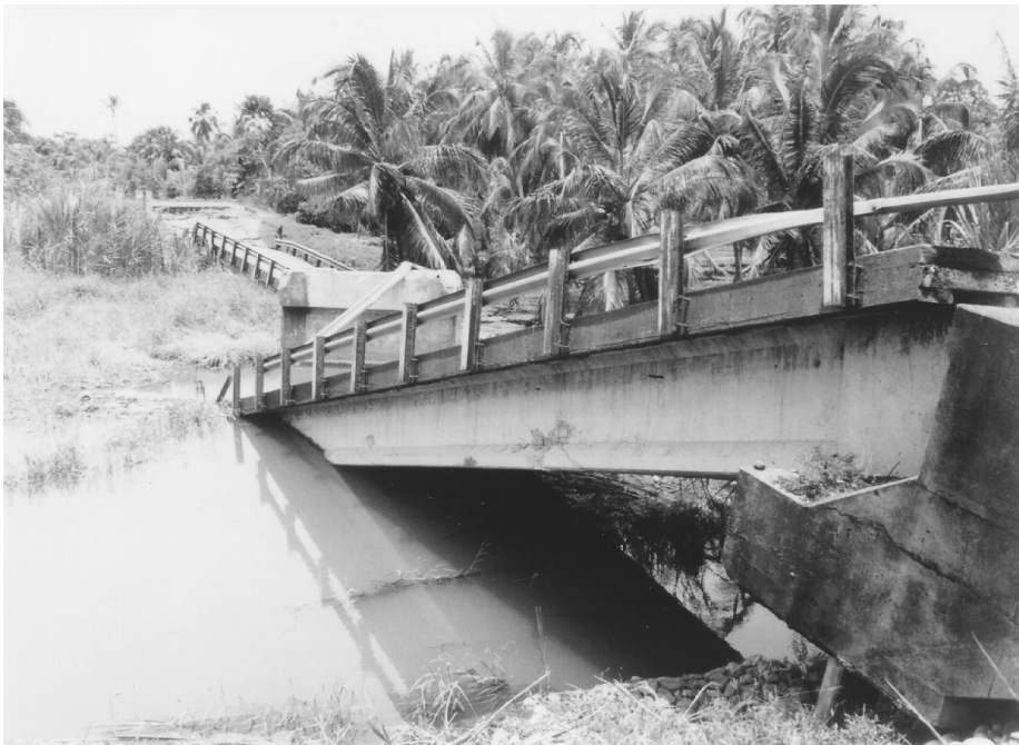
FIGURE 2.9 Rio Bananito Bridge collapse in the 1991 Costa Rica earthquake. (Source: EERI, Earthquake Spectra , Special Suppl. to Vol. 7, 1991.)
