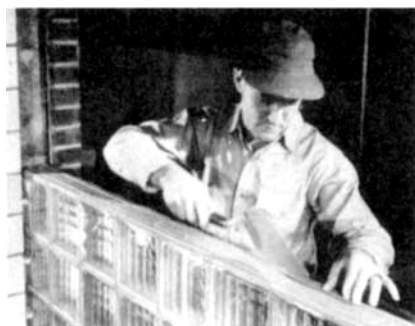
FIGURE 11.15 (Top left) First step in installation of a glass-block panel is to coat the sill with an asphalt emulsion to allow for movement due to temperature changes. Continuous expansion strips are installed at side and head jambs. (Top right) Blocks are set with full mortar joints. (Bottom left) Welded-wire ties are embedded in the mortar to reinforce the panel. (Bottom right) After all the blocks are placed, joints tooled to a smooth, concave finish, and the edges of the panel calked, the blocks are cleaned.
