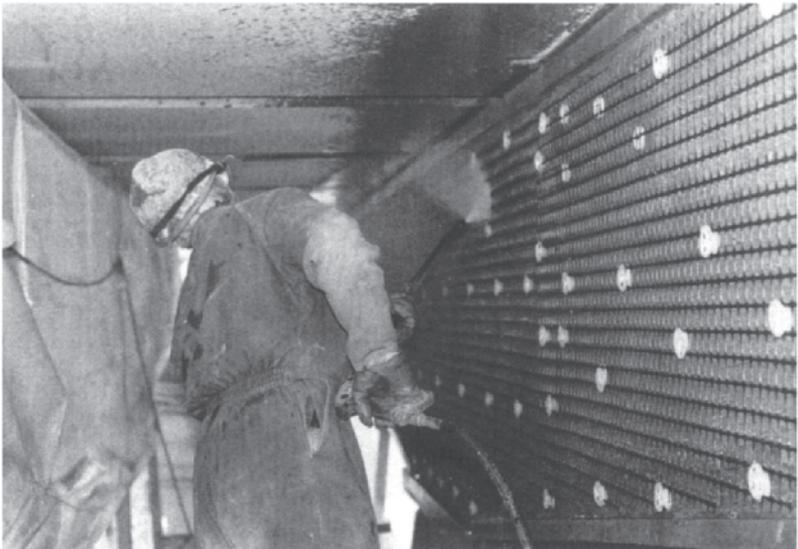
*Fig. 9.22. Polypropylene grid reinforcement for cover concrete. The plate shows the repaired concrete face being saturated prior to the spraying of an extra thickness of cover concrete. The grid is fixed with nylon spacer studs.*
