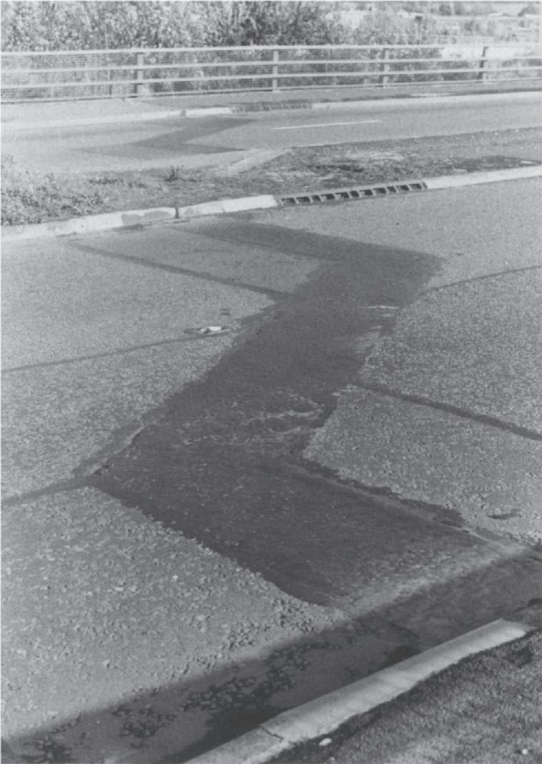
*Fig. 9.7. Bridging joint with severe skew. This deck end has a stepped plan alignment. The original joint failed and was replaced with rubberised bitumen, together with patch repairs to the adjacent asphalt.*
