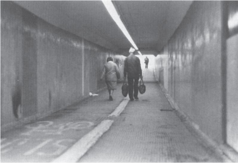
*Fig. 9.19. Early pedestrian subway. Because of its length, this mid-1960s subway was built 600 mm wider than the standards then in force. It has been converted recently to provide a cycleway.*
