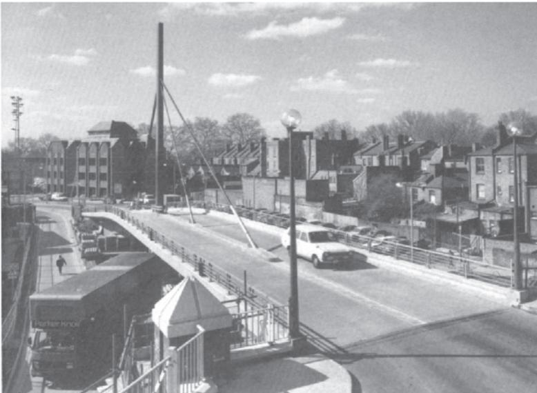
*Fig. 7.1. Cable-stayed lightweight aggregate bridge at the Baling Broadway Centre, London.*
