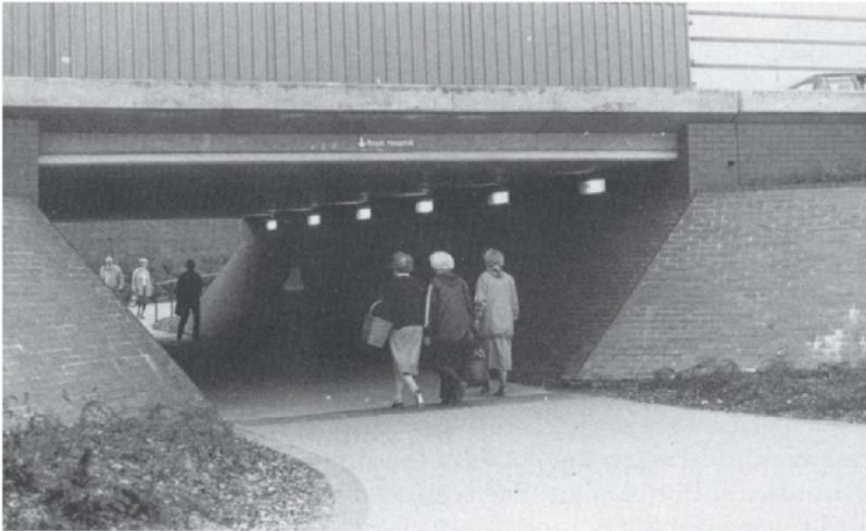
*Fig. 9.20. A pedestrian subway becomes a small bridge. Subway of the mid-1980s, having wide walkway, sloping brick-faced abutments, lights beyond the reasonable reach of vandals.*
