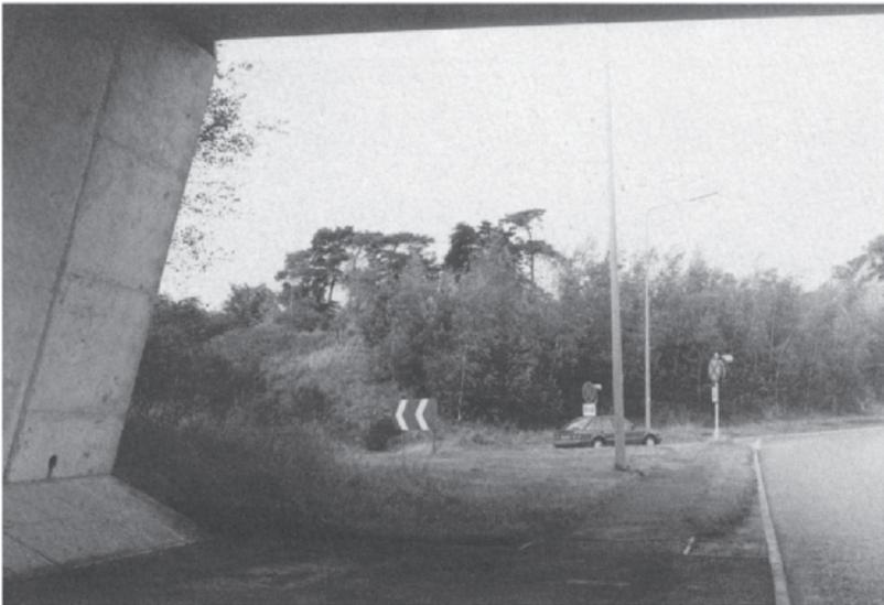
*Fig. 9.21. Inclined abutment. This particular span is wider than necessary. Full advantage of the potential sight-line is not achieved because the toe of the approach embankment spreads too far, amenity planting is too near to the abutment, and the horticultural maintenance stops short of the ideal standards for which the abutment was designed.*
