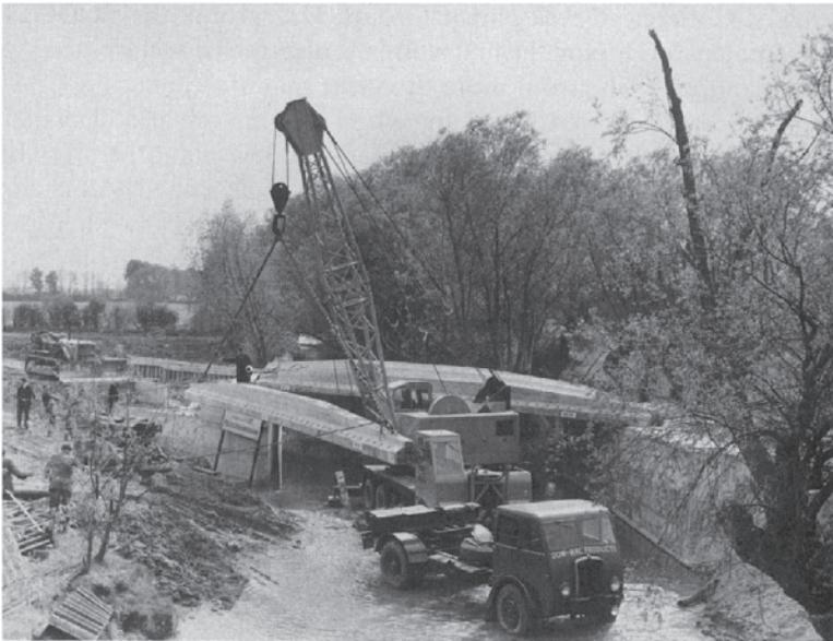
*Fig. 8.7. Early bridge with precast inverted T-type beams.*
