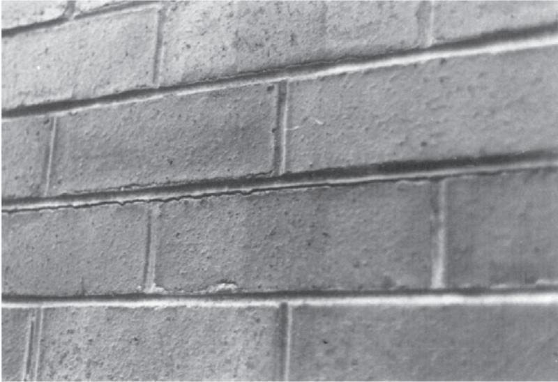
*Fig. 9.23. Cracked facing brickwork, showing a horizontal crack in the joint of integral facing brickwork at the level of concrete backing lift.*
