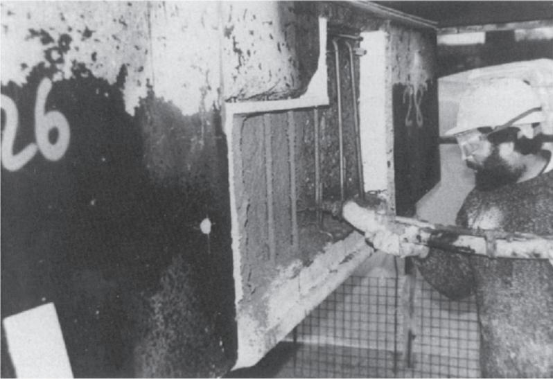
*Fig. 9.30. Alternate panel repairs. Panel 27 is being repaired except for a portion below the bearing which will follow later. Panels 26 and 28 will be repaired when 27 has cured.*
