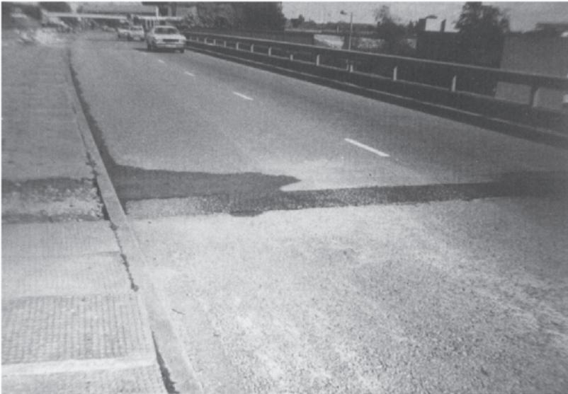
*Fig. 9.5. Dam caused by bridging joint. Subsurface water, mostly under central reservation, emerging on surface adjacent to rubberised bitumen joint.*
