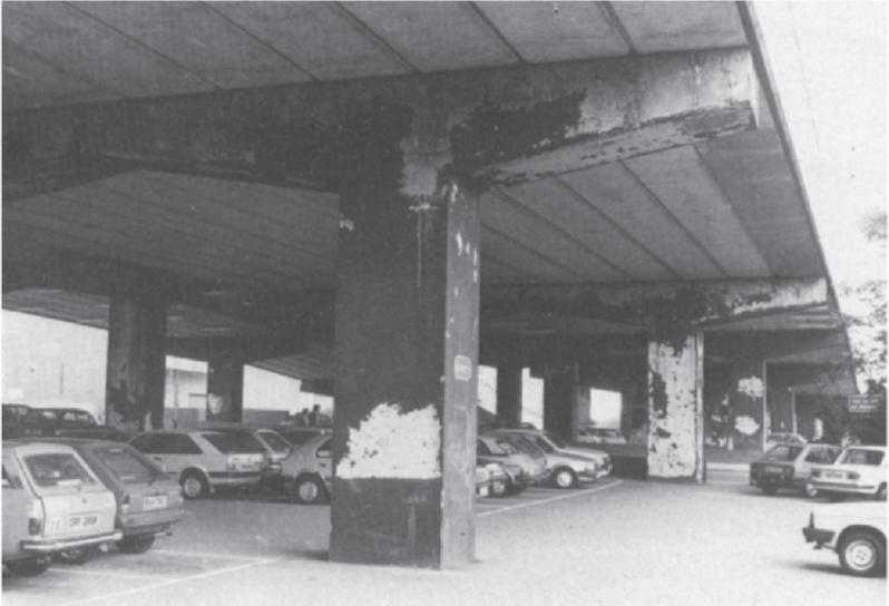
*Fig. 9.24. Neglected decorative painting of viaduct piers. Originally coloured black, contrasting dramatically with the white exposed aggregate fascias, these viaduct piers now have an untidy, neglected appearance.*
