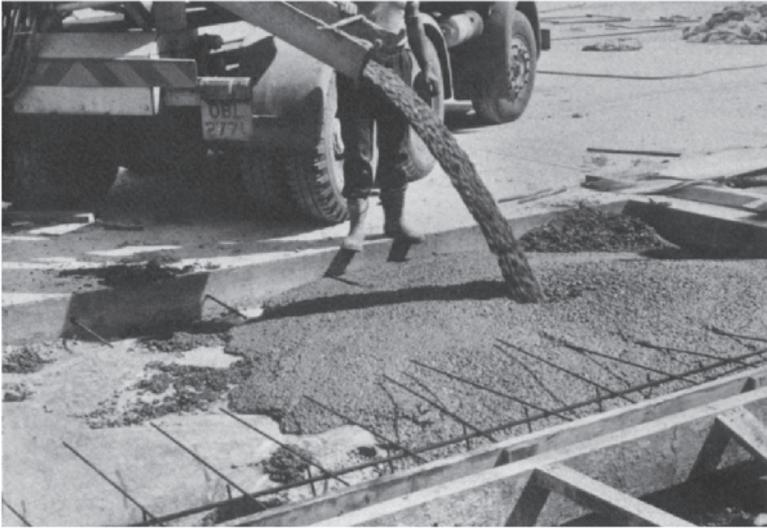
*Fig. 7.7. Flowing concrete.*
