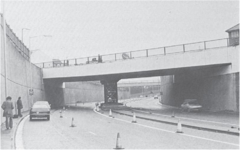
*Fig. 3.2. 45°, voided reinforced concrete slab bridge with temporary central support.*
