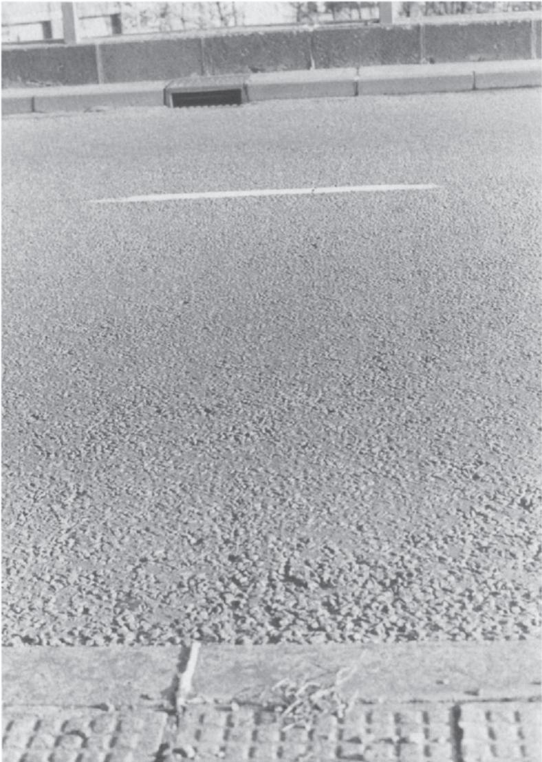
*Fig. 9.3. Successful buried joint. The position of the joint is marked by the sealant in the kerbs and the crack in the thermoplastic white line. After 21 years of medium volumes of mainly light traffic, the asphalt remains uncracked, although there is some leakage of water. This is a viaduct fixed end joint, having dynamic rotational movements only.*
