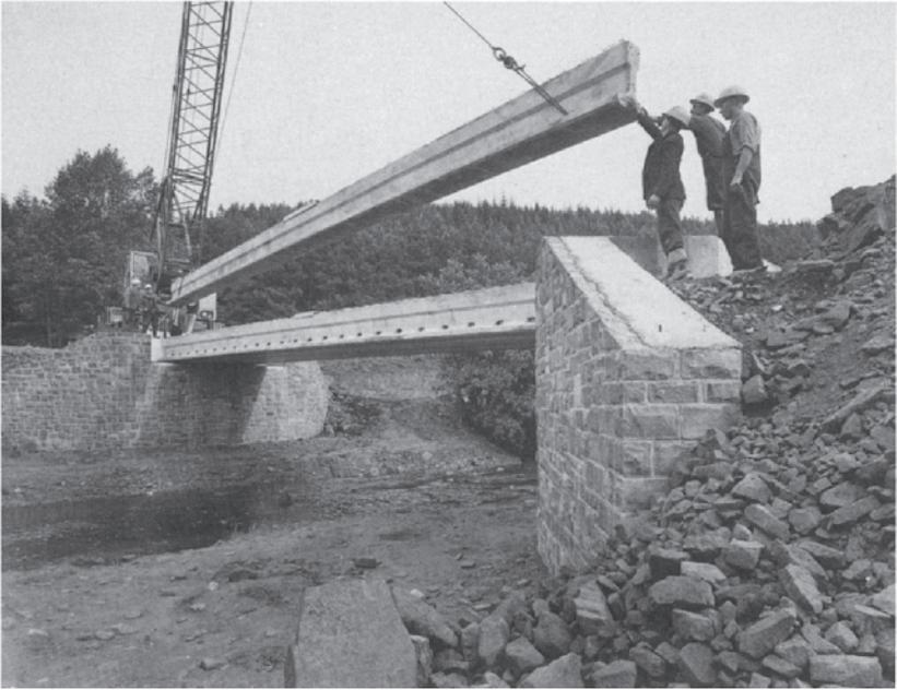
*Fig. 8.9. Lightweight concrete inverted T bridge constructed in 1969.*
