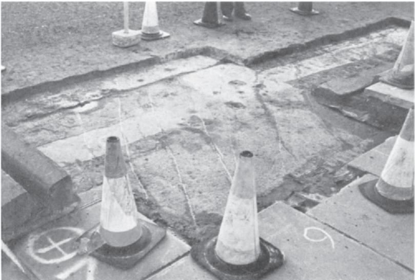
*Fig. 3.3. Top surface cracking in an obtuse corner (courtesy of Mersey side County Council).*
