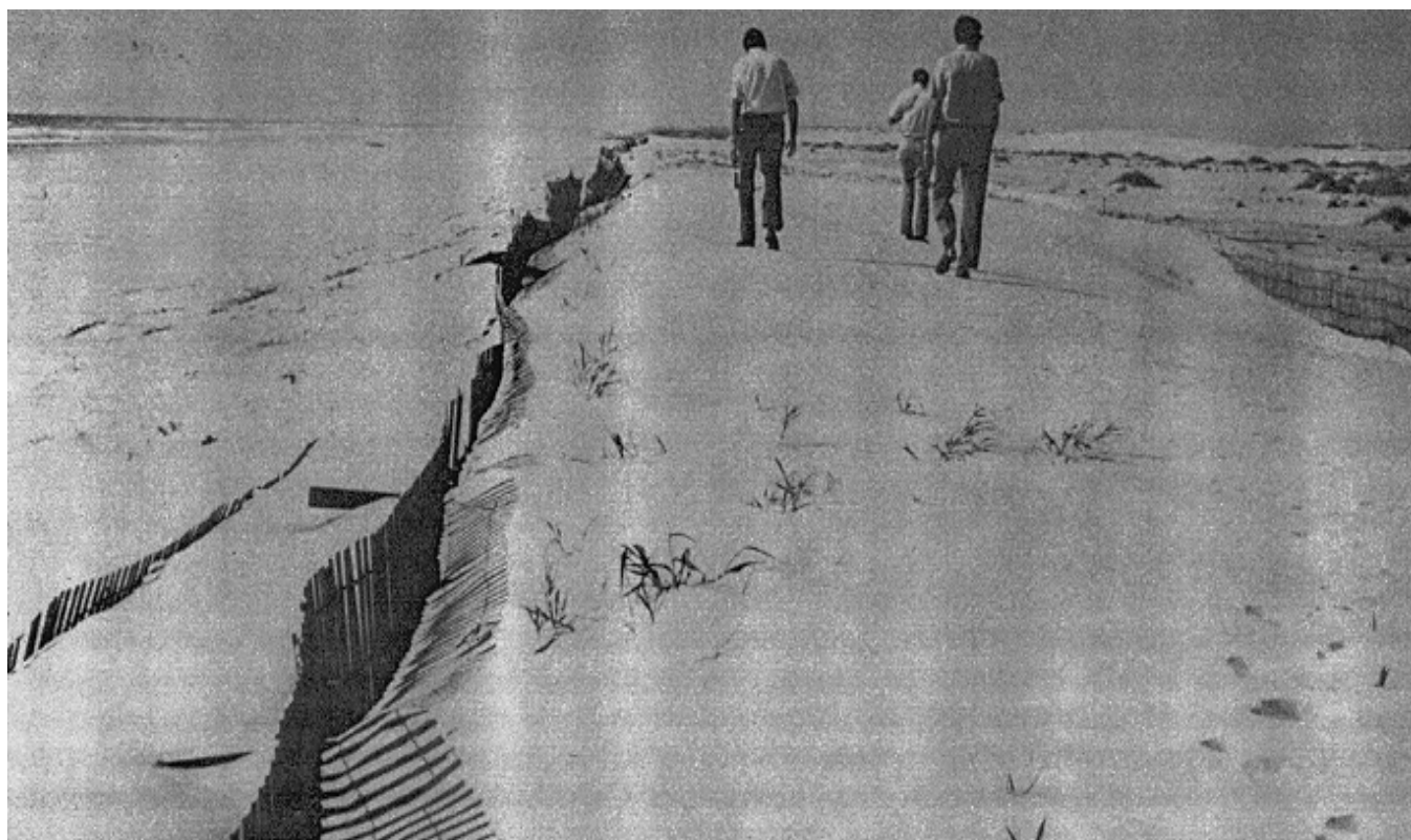
Figure 5-6. Snow-type sand fencing for dune stabilization at Padre Island, TX ( Shore Protection Manual (1984))
