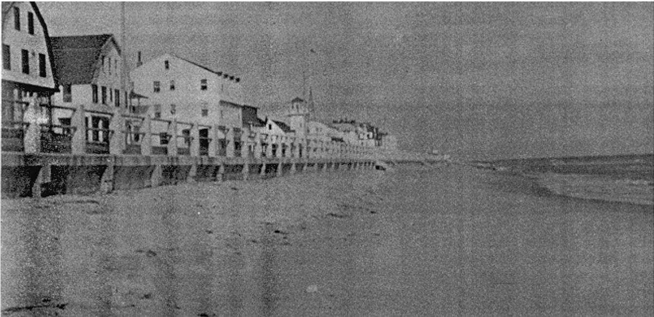
Figure 5-5. Concrete slab and king-pile bulkhead at Virginia Beach, VA ( Shore Protection Manual (1984))
