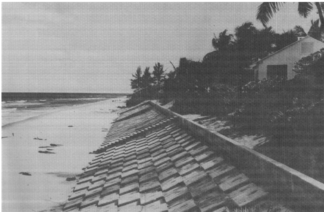
Figure 5-3. Concrete block revetment at Jupiter Island, FL ( Shore Protection Manual (1984))
