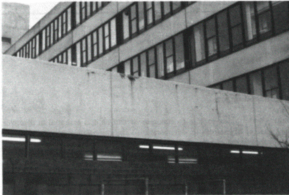
Fig. 3.1 Deterioration of repair to calcium-chloride-affected concrete after four years. Incorrect diagnosis and specification.
