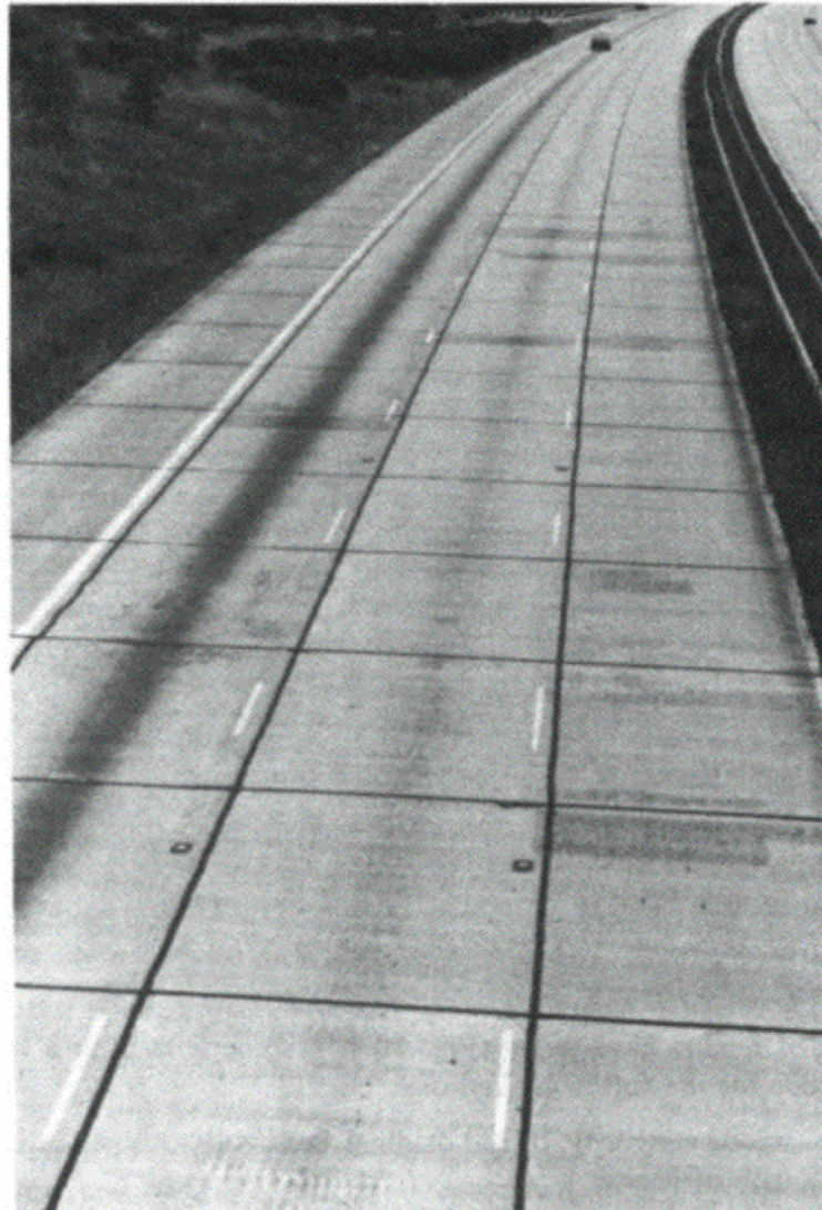
Fig. 10.10 Overhand sealing of joints.
