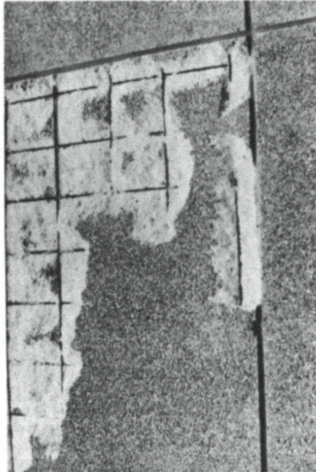
Fig. 9.14 Carbonation at Banbury Station.
