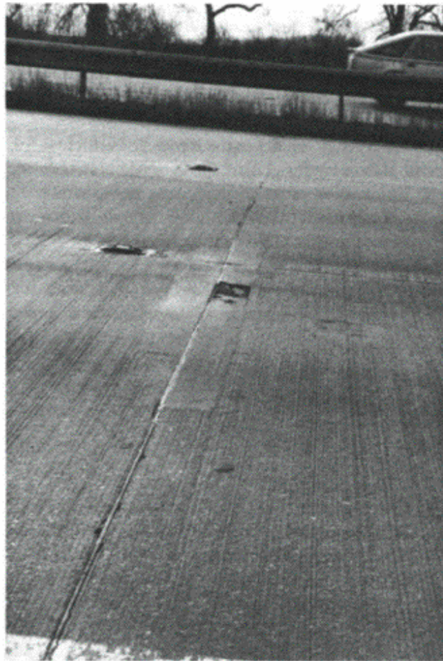
Fig. 10.12 Failed arris repair
