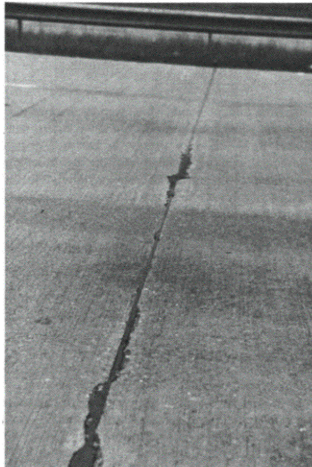
Figure 10.7 Spoiled joint.
