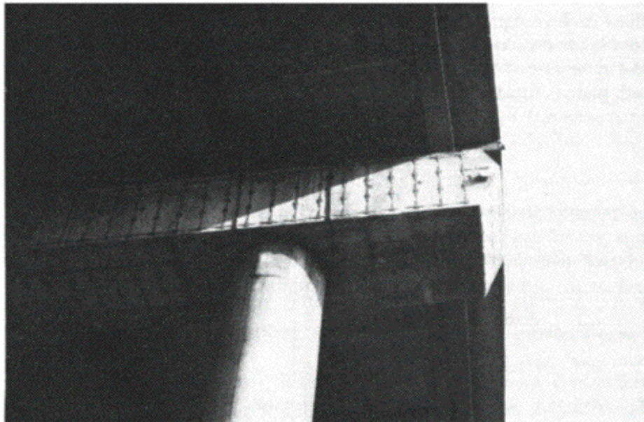
Fig. 5.11 Ceramic plates fixed to bridge beam (courtesy of Ebonex Technologies Inc., California, USA).
