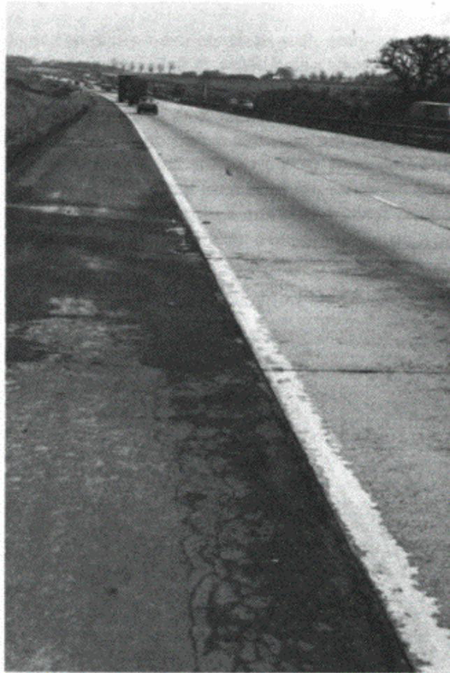
Fig. 10.5 Seepage of water over the hard shoulder from beneath the concrete carriageway.
