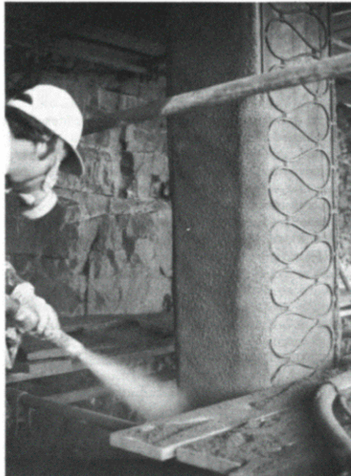
Fig. 5.6 Fixed anode cover coat on bridge column (courtesy of Raychem Ltd, Swindon, Wilts.).
