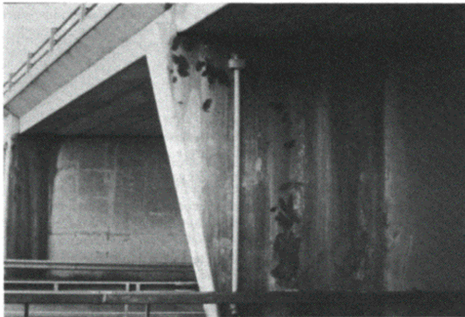
Fig. 3.2 Failure of drainage system on bridge pier/abutment.
