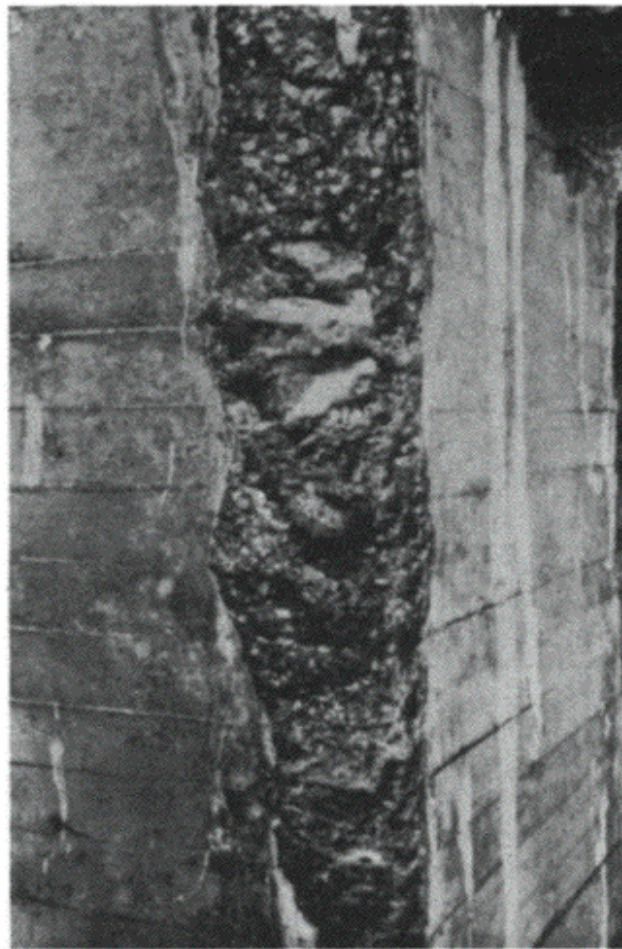
Fig. 9.16 Frost attack, Glenfinnon Viaduct.
