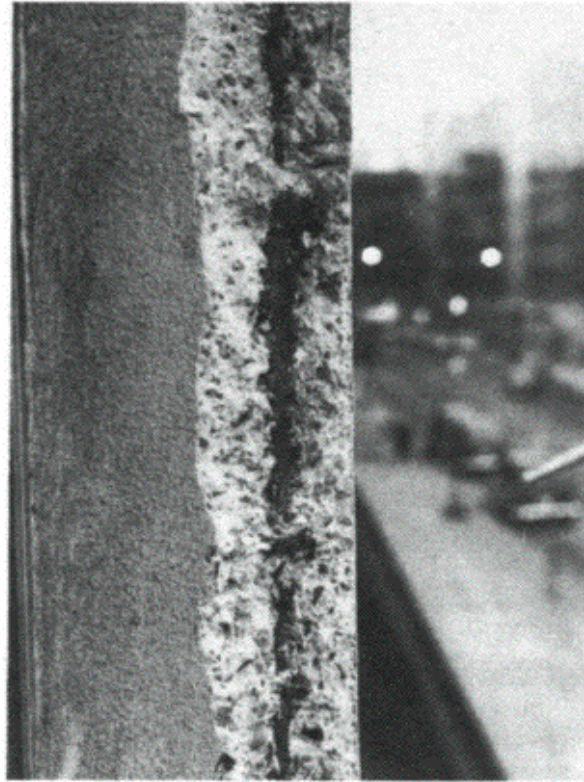
Fig. 9.13 Repair failure on multistorey office block, London.
