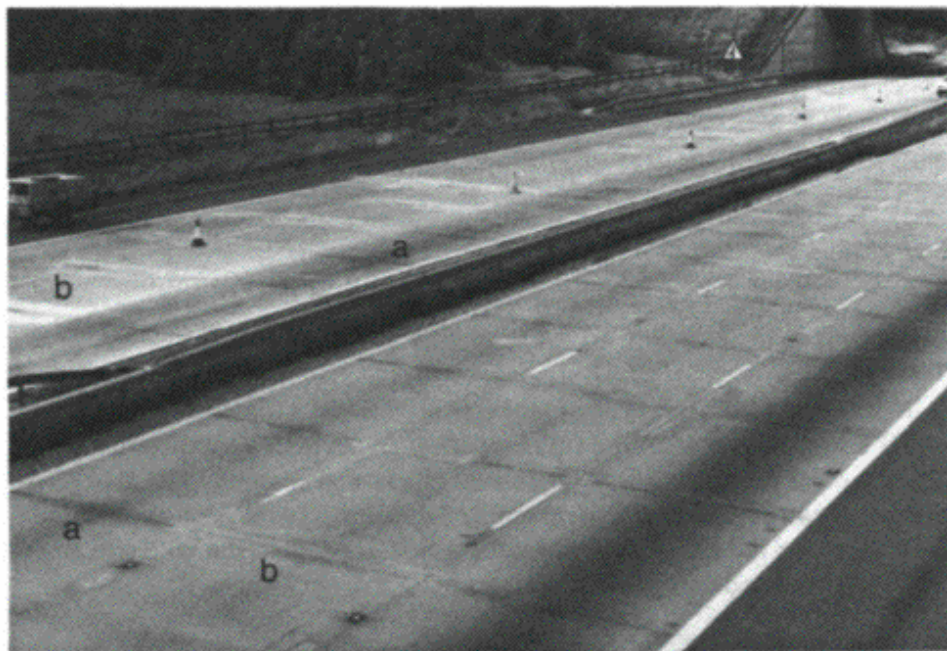
Fig. 10.6 Slip-formed concrete pavement: a, poorly compacted permeable concrete at transverse joints in outer lanes; b, joint aris repairs to most transverse joints in centre and inner lanes.
