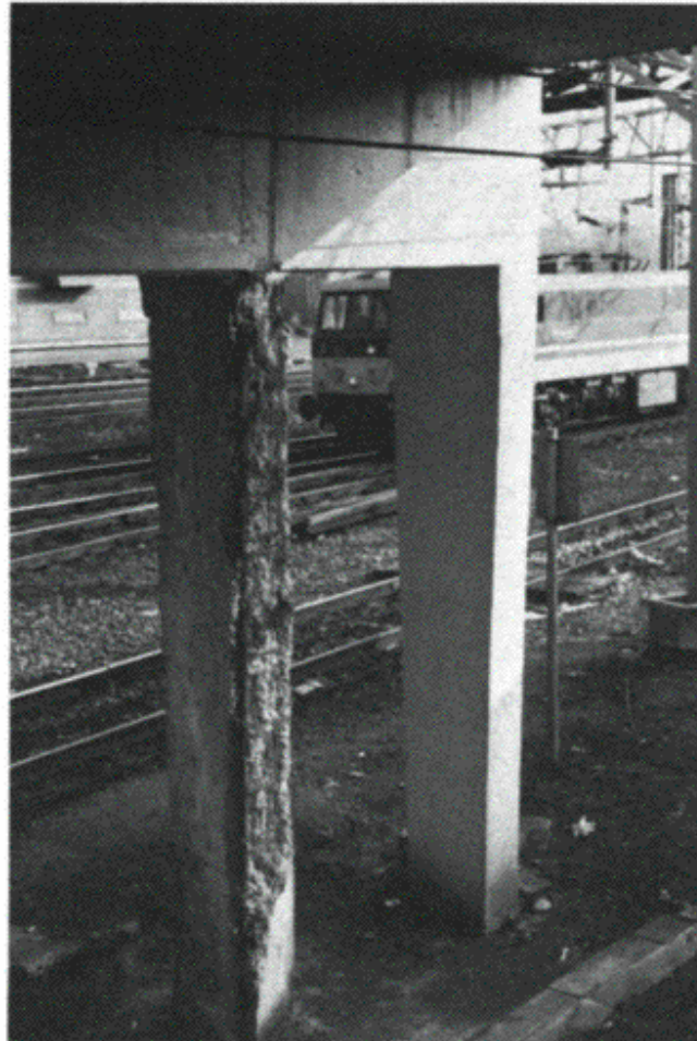
Fig. 9.9 Repaired column, Stafford Bridge.
