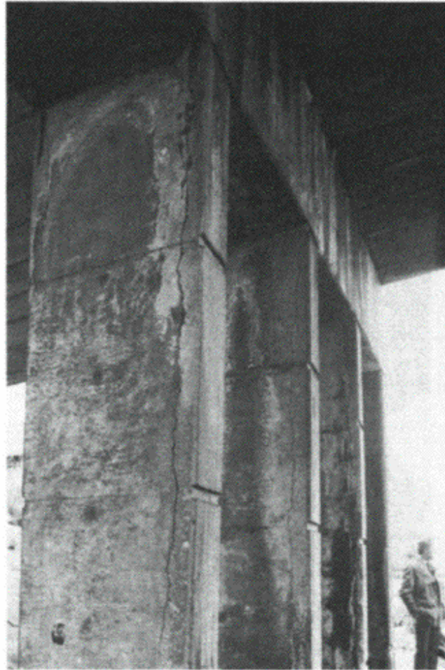
Fig. 9.5 Evidence of water seepage and spalling of columns, Stafford Bridge.
