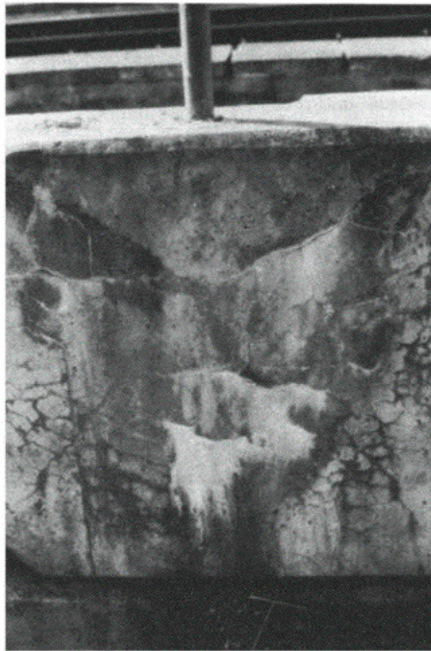
Fig. 9.17 Bridge parapet suffering from alkali-silica reaction.
