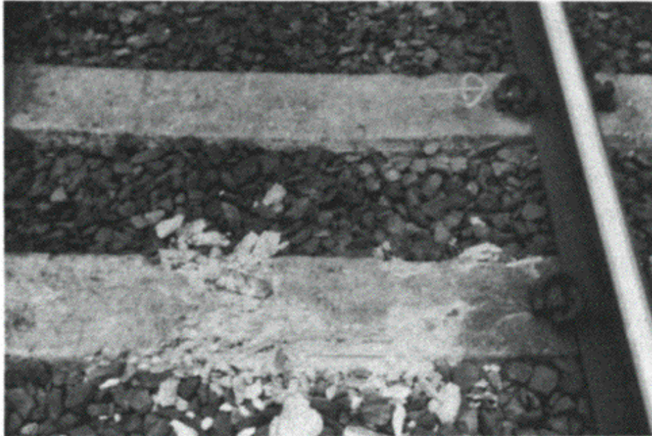
Fig. 9.15 Frost attack, prestressed concrete sleeper.
