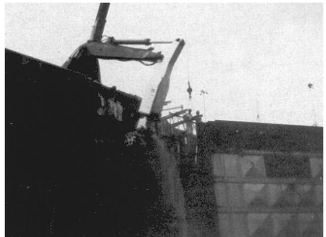
Figure 5-11. Rotary-head milling
