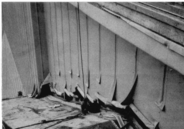
**Figure 8-62. Installation of geocomposite, Pracana Dam**
