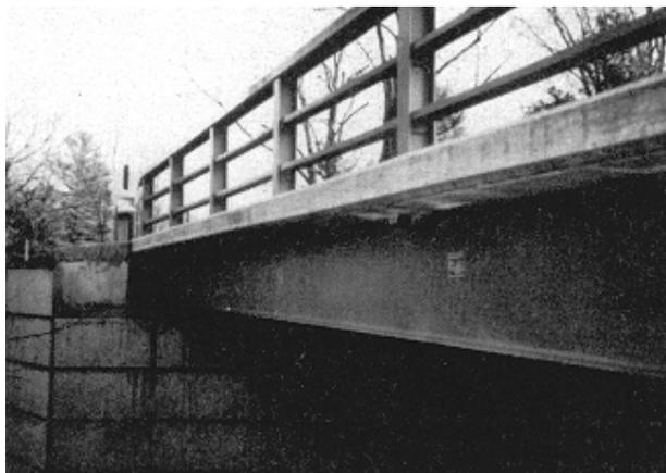
**Figure 8-53. Precast abutment and deck units, Ulsterville Bridge**
