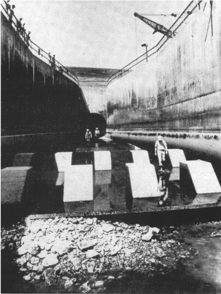
**Figure 8-30. Stilling basin dewatered for inspection, Pomona Dam**
