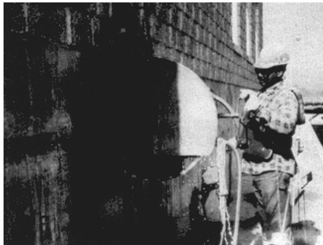
**Figure 5-3. Diamond-blade saw**
