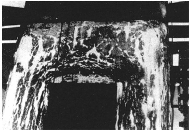
**Figure 2-24. Efflorescence**
