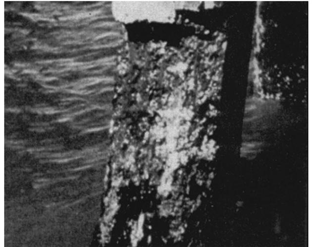
**Figure 2-13. Disintegration of concrete caused by exposure to acidic water**
